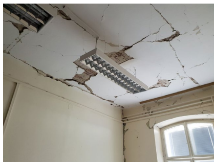
Earthquake damage inside. The earthquake damaged office areas in the DHMZ building.
